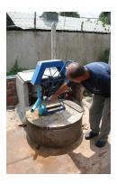
Rainwater Harvesting Tank with Rovai Pump with a well beside it.
