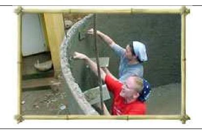
A reliable source of clean drinking water is also needed at schools. Rainwater harvesting tanks like the one pictured can be built on site for about US\$1500.
